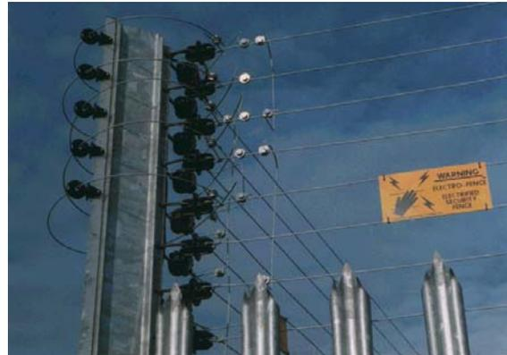
The Electro-fence™ system can be broken down into zones so that the Controller immediately recognises the attempted entry location. In the event of power failure, uninterrupted power is supplied by battery back-up system.
