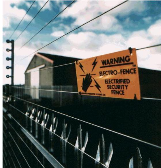
All Electro-fence™ Controllers have been manufactured to exceed European standards: EN61011/1; EN61011/2. Electric fence controllers have an impeccable safety record. The high voltage pulse is of less than one thousandth of a second in duration.
